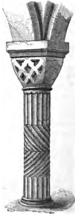
31. Crypt, Canterbury, A.D. 1110. Norman capital, with carving commenced and left unfinished.
